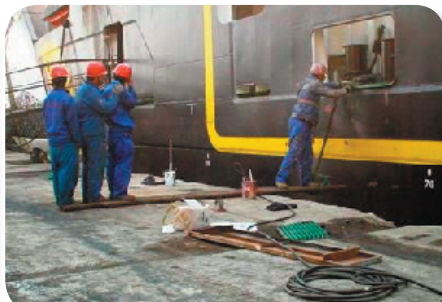
Osha approved scaffolding
